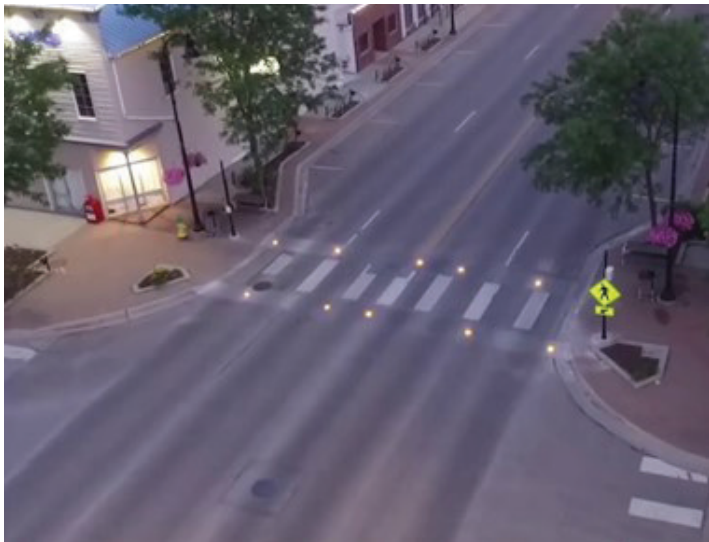
FIGURE 5: IN-PAVEMENT CROSSWALK LIGHTING IN PAPILLION
