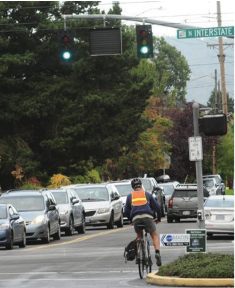
FIGURE 9: DETECTION CONFIRMATION SYSTEM IN PORTLAND
