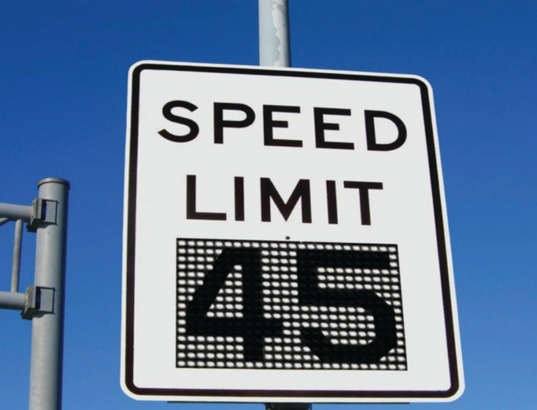
FIGURE 13: VARIABLE SPEED LIMIT SIGN
