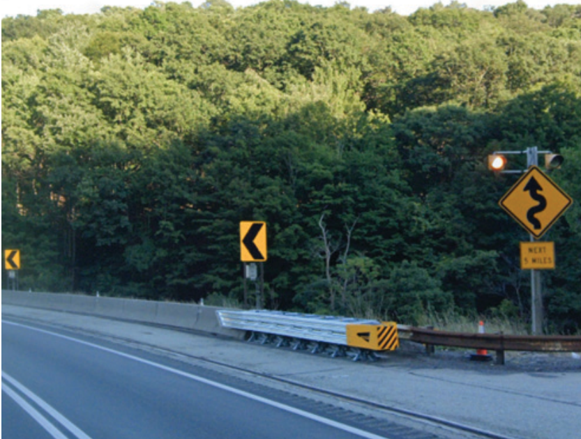
FIGURE 11: DYNAMIC CURVE WARNING SYSTEM ALONG PENNSYLVANIA TURNPIKE
