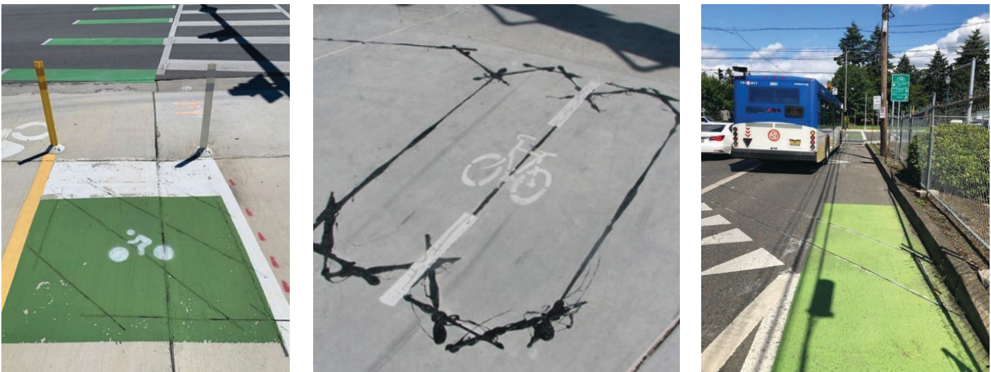
Type D Loop in Huntsville, Alabama (left): Type Q Loop in San Luis Obispo, California (middle): Parallelogram Loop Detector in Portland, Oregon (right).
