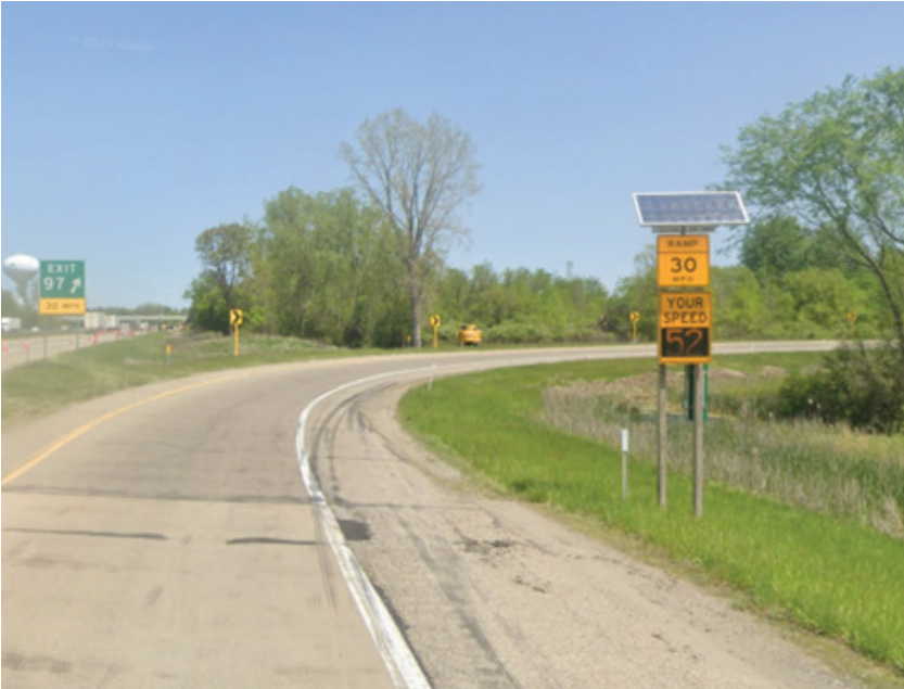
FIGURE 10: DYNAMIC SPEED FEEDBACK SIGN WEST OF LANSING
