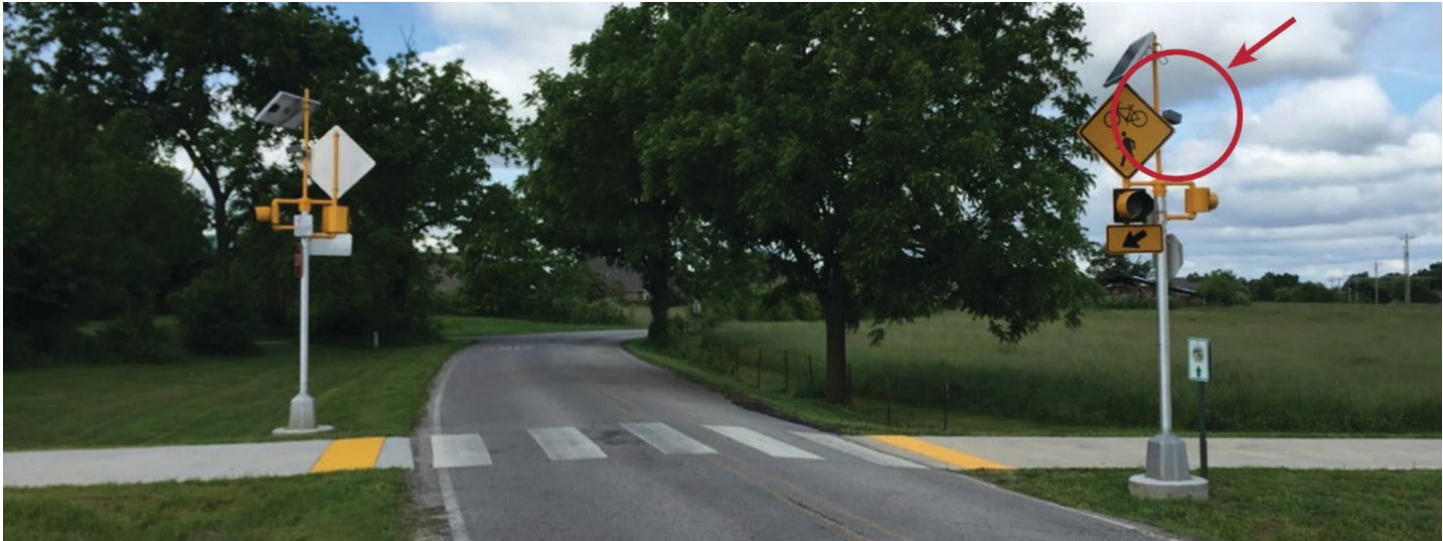
FIGURE 8: MICROWAVE DETECTION ALONG RAZORBACK GREENWAY TRAIL IN ARKANSAS
